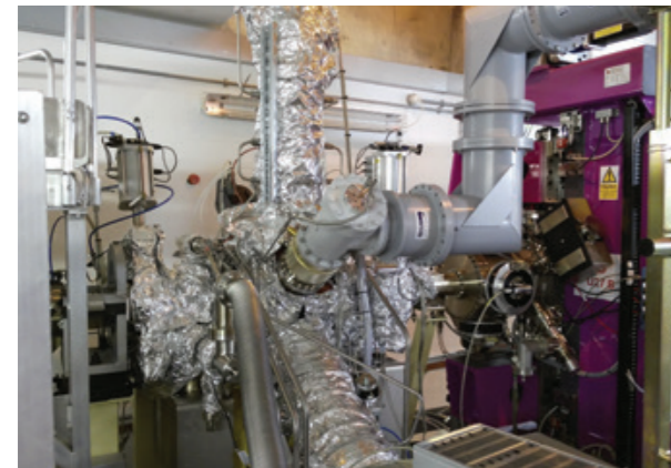
Figure 2: The cavities are installed in straights 16 and 18, on either side of straight 17 which hosts the two superconducting cavities.
