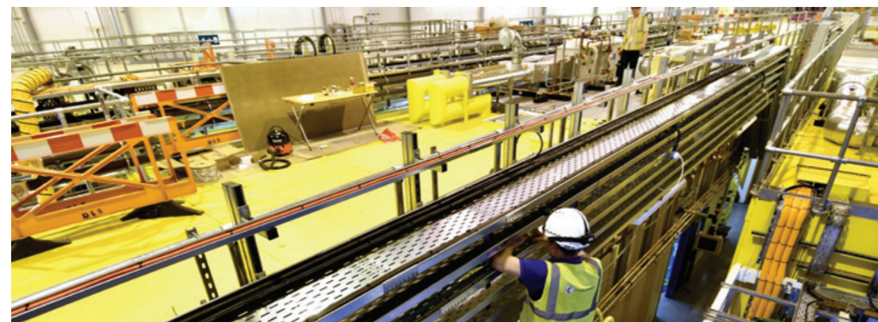
Figure 1: Construction of the hutches nearing completion for DIAD.
