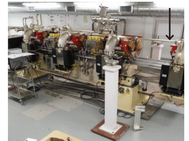
Figure 5: Replacement girder under construction; the arrow indicates the position of the 'missing sextupole' and the new narrow gap vacuum vessel where the DIAD mini-wiggler will be installed.
